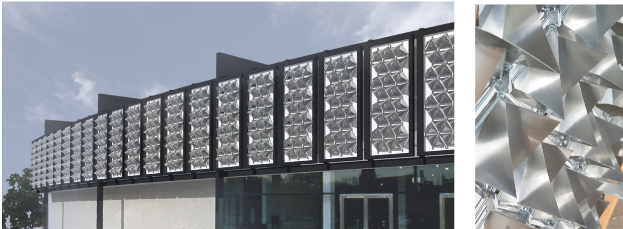
Figure 1 : A transformable shading system proposed for the Museum of Fine Arts in Houston.
